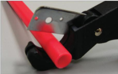
1. Cut PEX tubing square, leaving a clean, even edge. Remove any burrs.
